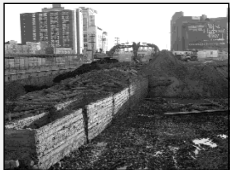
The discovery: A structure almost 40 metres long built of 28-centimetre square white-pine timbers, still held together with wooden dowels and iron spikes
