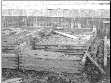
The discovery: A structure almost 40 metres long built of 28-centimetre square white-pine timbers, still held together with wooden dowels and iron spikes
